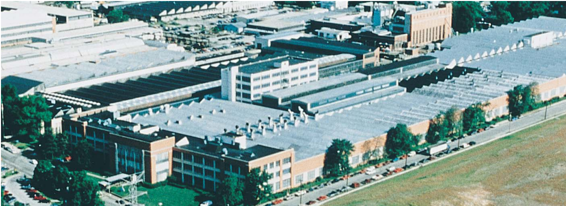
Innovative coupling of steam generation and absorption cooling technologies created financial opportunities at Cincinnati Milacron's 1.5 million ft 2 (139 350 m 2 ) headquarters complex.
