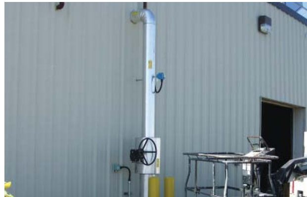
Tie-In at Main Plant
