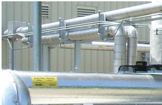
Tie-In at Water Reclamation Plant
