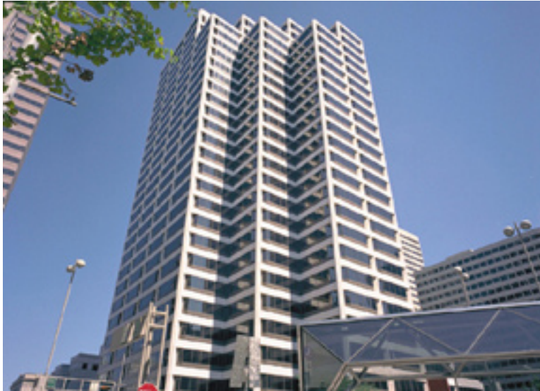
PNC Bank Data Processing Center
