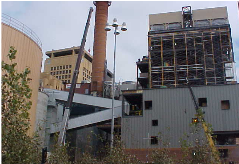
Cogeneration Plant (under construction)
