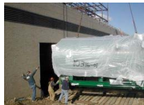
Rigging 800 HP Firetube Boiler
